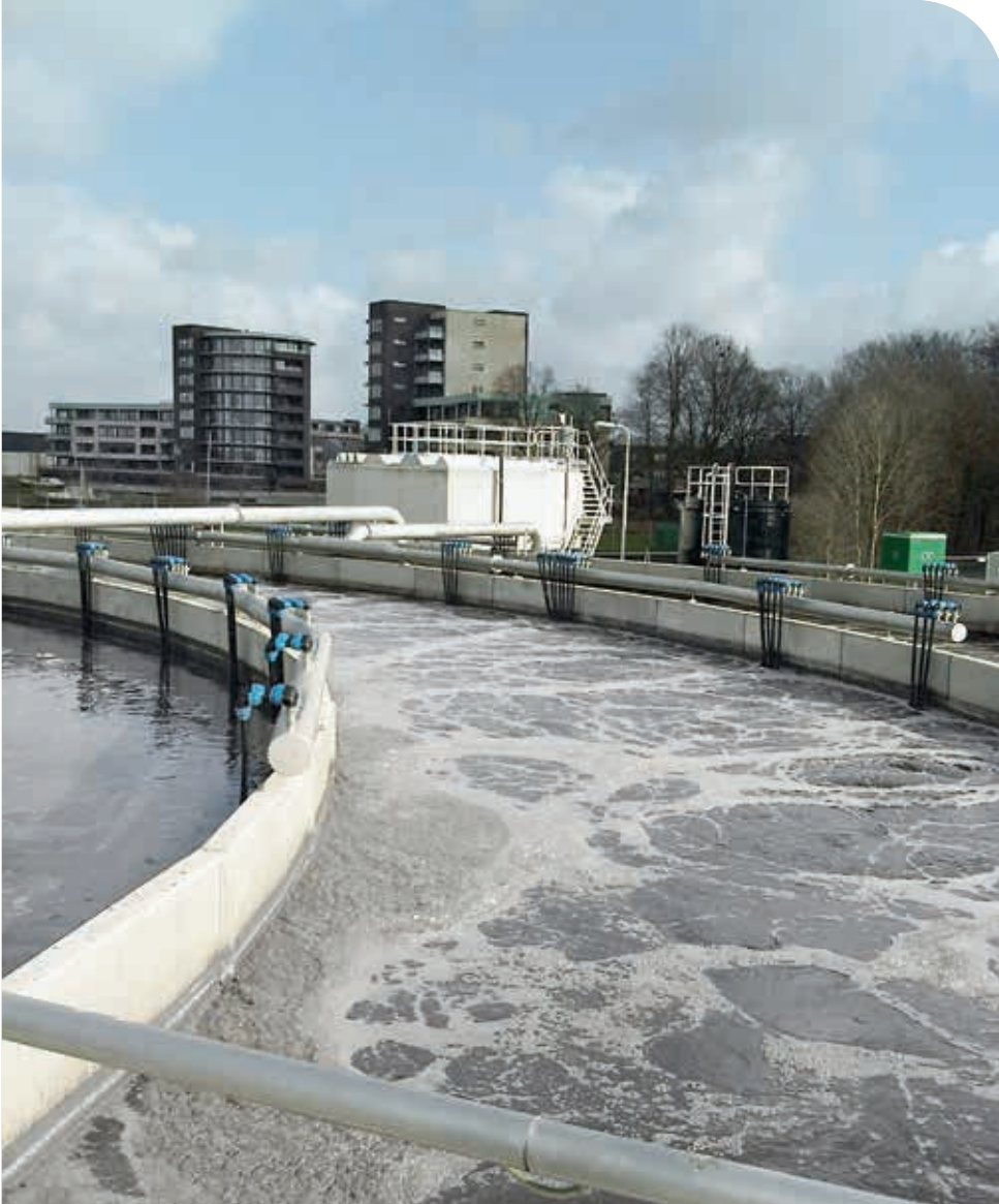
Wastewater treatment plant Steenwijk, Netherlands
